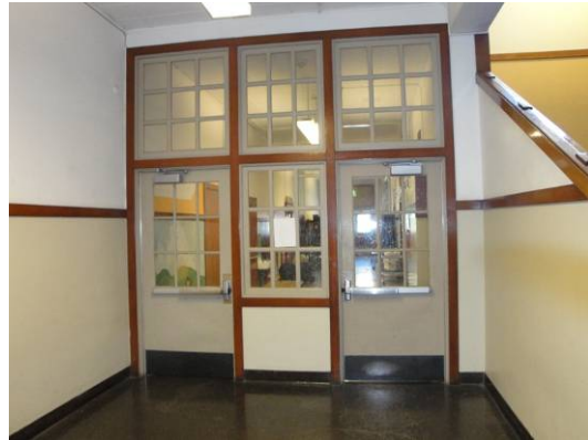
Stairwell entry hall
