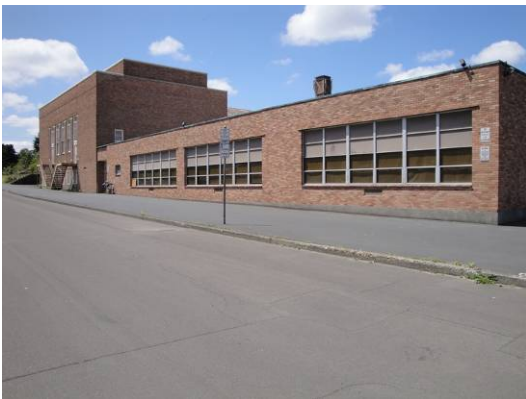
East elevation addition
