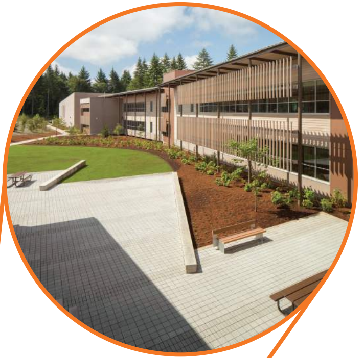
Example of a courtyard Sandy High School, IBI Group
