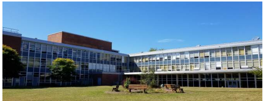
Exterior photo: Courtyard
