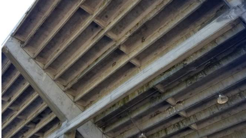
Exterior photo: Underside of stadium seating at track and field
