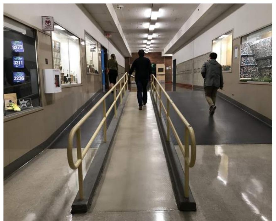
Interior Photo: ADA ramp modification
