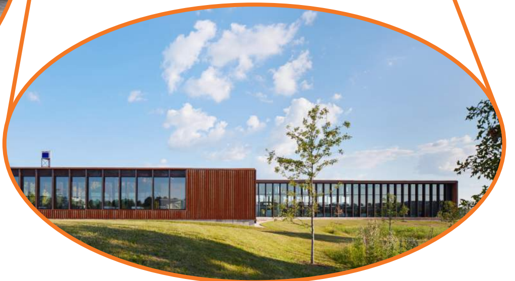
Example of exterior materials and building relationship to the landscape Trumpf Smart Factory Chicago, Barkow Leibinger
