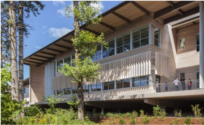
Example of the building connecting with the landscape Sandy High School, IBI Group
