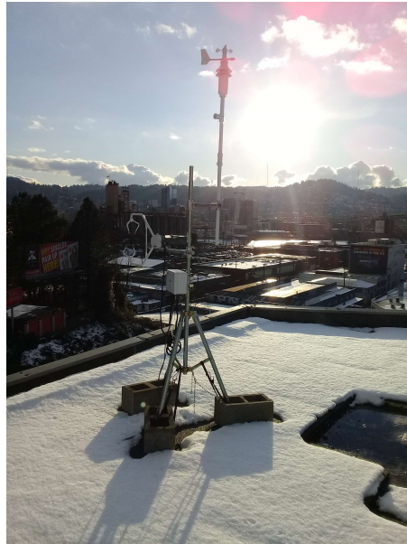
Figure 3. Installation of weather station on HTMS rooftop.
